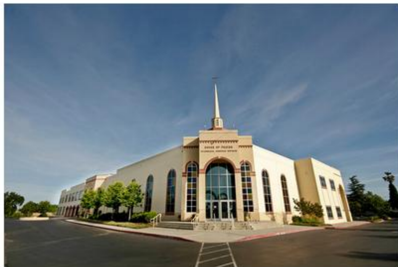
The main east entrance to the central worship hall.
